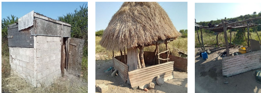
Figure 6-3 – Diverse Selection of Impacted Auxiliary Structures
